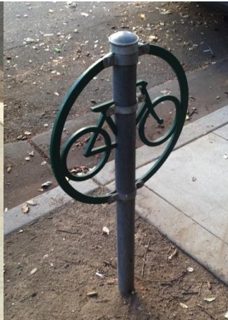
Meter post conversions. Over 100 installed.
