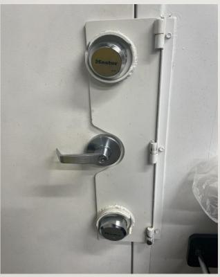
1010.1.3 Door Opening Force doors shall not exceed 5 pounds to open interior doors. The forces to operate door hardware shall not exceed 15 pounds of force, 30 pounds to set in motion and 15 pounds to full open"
