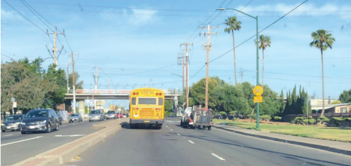
Figure 1- Existing Florin Road and Light Rail Overcrossing
