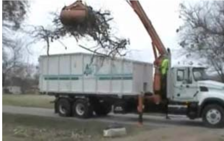
Figure 4 – Boom Truck Approach for Collecting LITS
