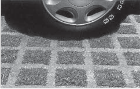
Alternative surfaces such as grass pavers keep stormwater runoff on-site and reduce heat production.
