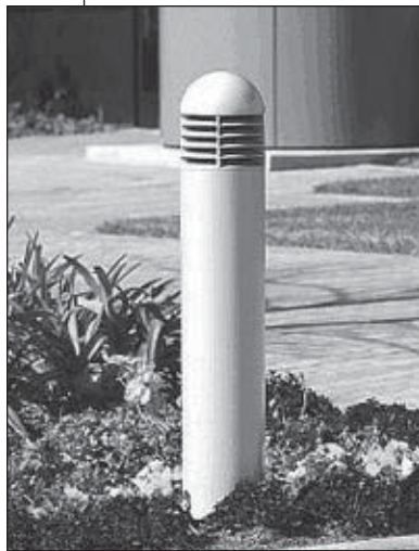
Pedestrian-scaled bollard lighting
