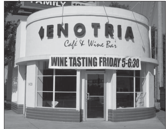
Renovated corner entry on Del Paso Boulevard
