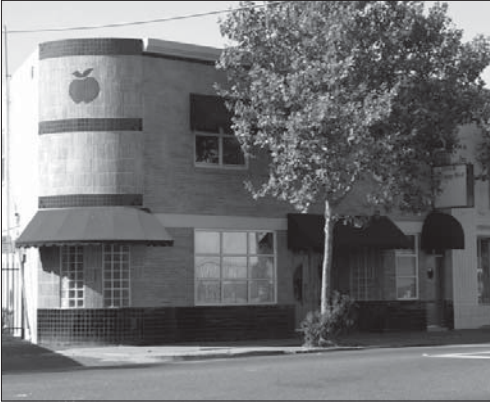
Renovated Streamline Moderne building
