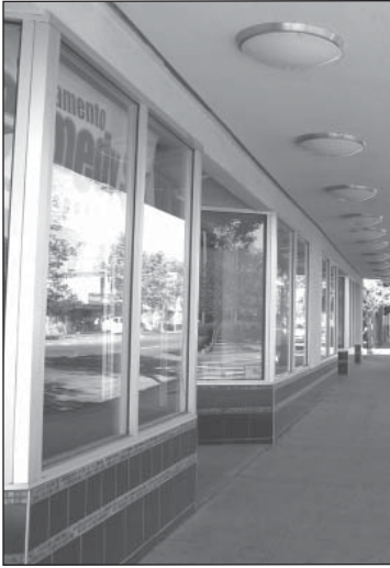
A commercial facade lined with transparent glass is highly desirable.
