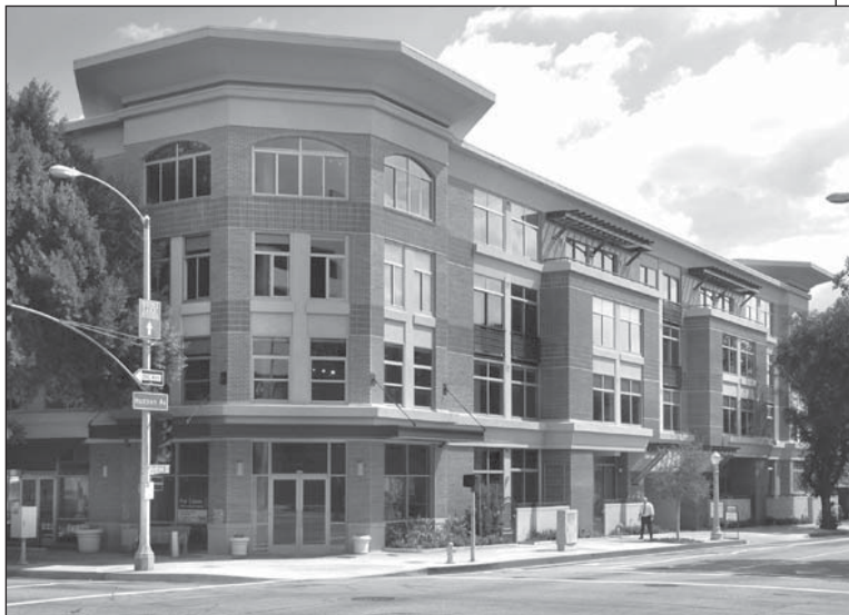
This mixed use building has a strong corner treatment, a clearly defined base, and an articulated facade.
