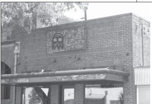
Typical flat commercial roof
