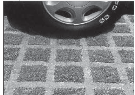
Alternative surfaces such as grass pavers keep stormwater runoff on-site and reduce heat production.
