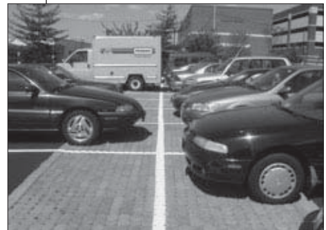
Modular pavers are another attractive alternative that helps to keep stormwater runoff onsite.
