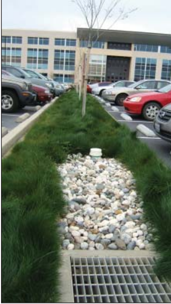
Bio-swales collect stormwater runoff and improve run-off water quality.
