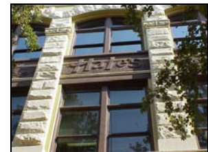
831 K Street Constructed 1881
