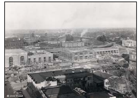
Image & photo courtesy of SAMCC
