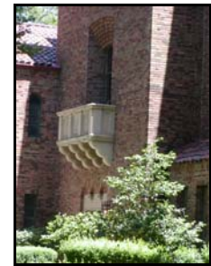
Juliet Balcony - Memorial Auditorium
