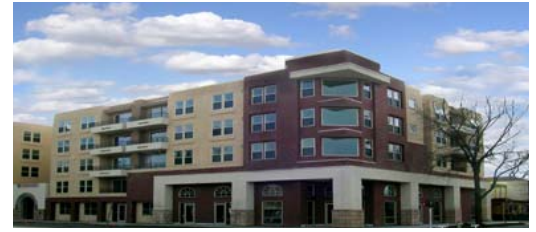
The St. Anton Building, above, is an example of a commercial product type. Photo courtesy St. Anton Partners.
