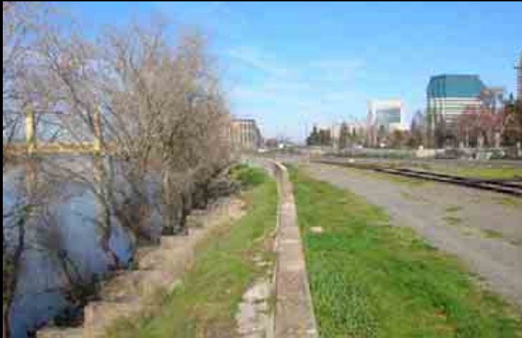
Levee facing North
