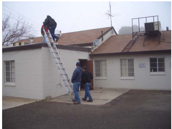
Deferred Maintenance Project Roof Replacement at Fire Station 57
