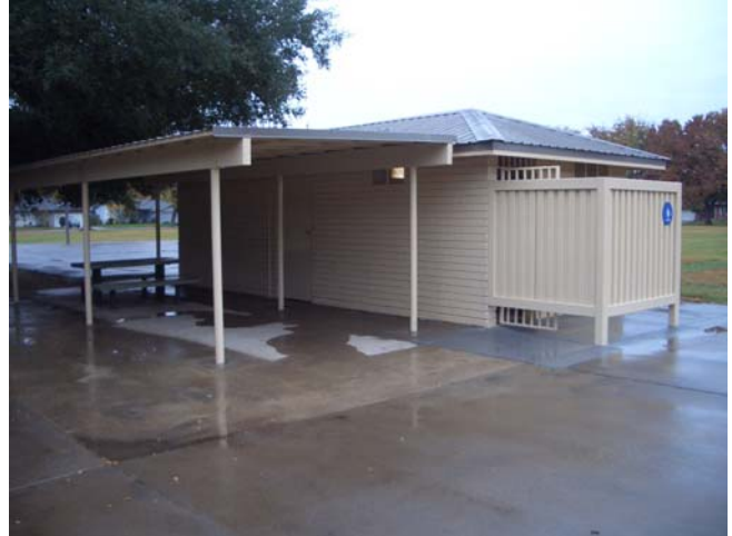
Lawrence Park Restroom Repair (after)
