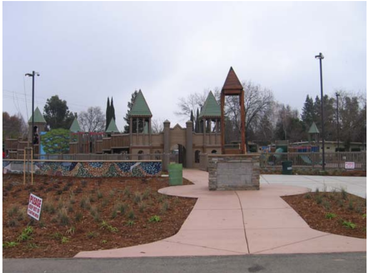
Fort Natomas at South Natomas Community Park Rebuild
