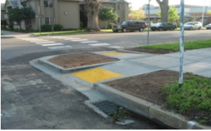
Curb Ramps with Truncated Domes
