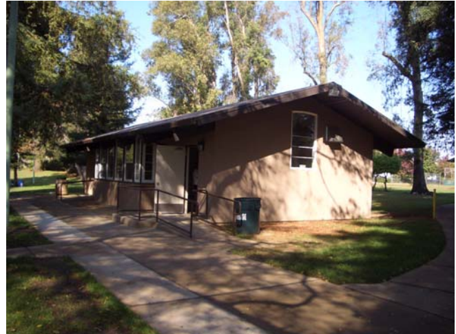
ADA Access to East Portal Park Restroom
