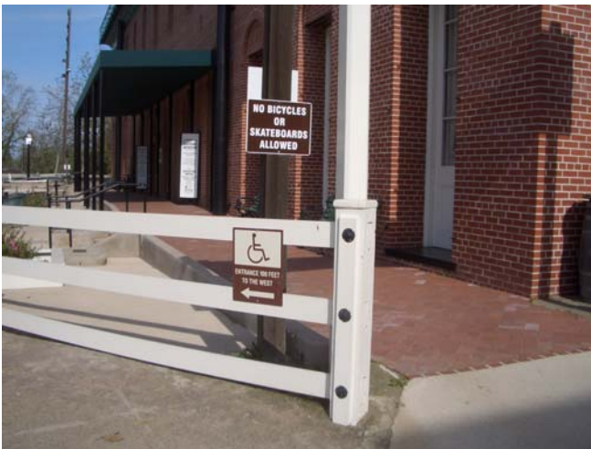
Old Sacramento Museum ADA Access
