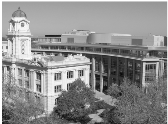
City of Sacramento – City Hall 2005
