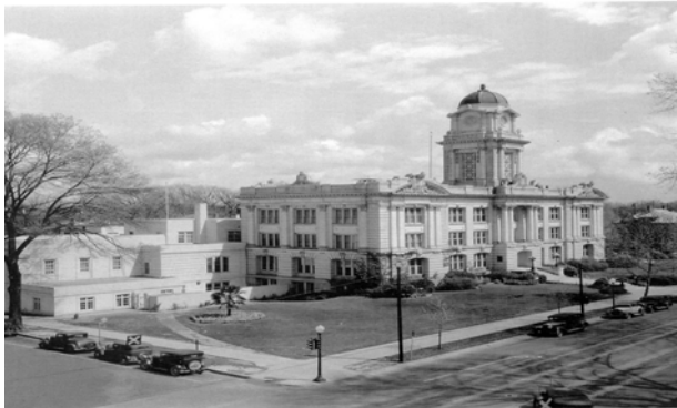
City of Sacramento – City Hall 1939
