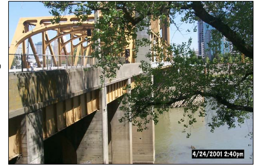
SOUTHWEST APPROACH FACING EAST
