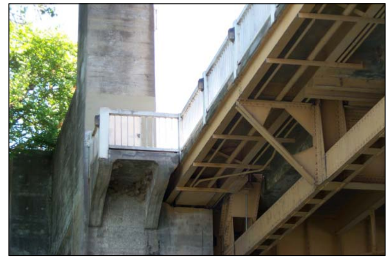
NORTHEAST CORNER LOOKING EAST
