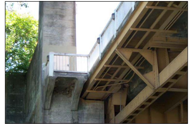
NORTHEAST CORNER LOOKING EAST
