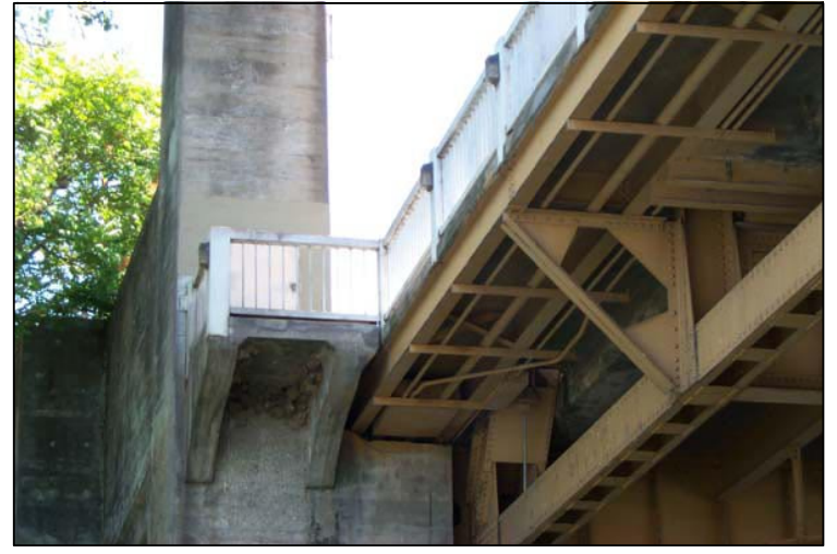
NORTHEAST CORNER LOOKING EAST
