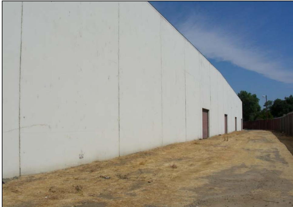
Photograph 34: Building 13, camera facing northwest, 08/29/2006.
