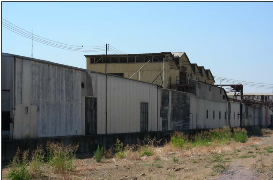
Photograph 5: Building 4, camera facing south, August 2006.
