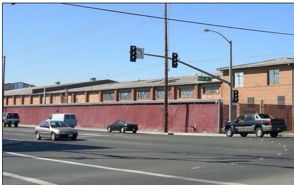
Photograph 5: Building 2, camera facing northwest along Richards Boulevard, 08/29/2006.
