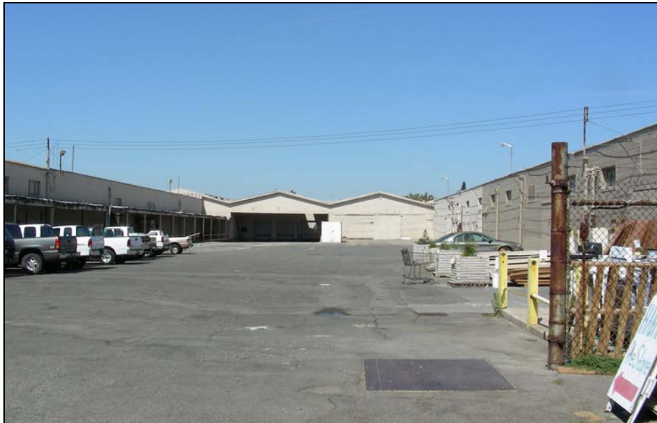
Photograph 6: Buildings 9, 6, 7 and 8 (left to right), camera facing west, August 2006.
