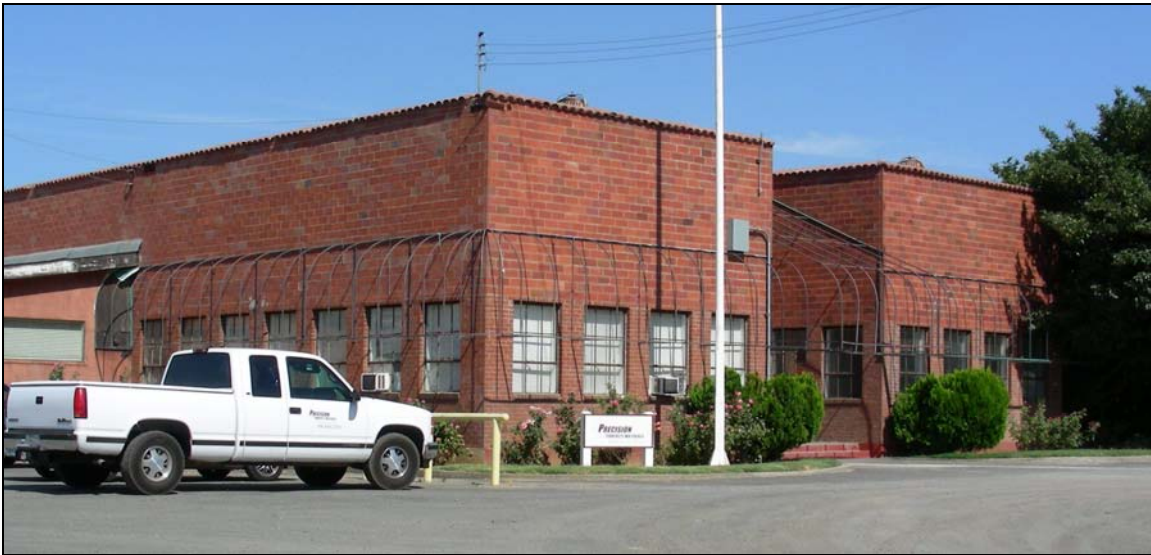
Photograph 7: Building 12, camera facing northwest, August 2006.
