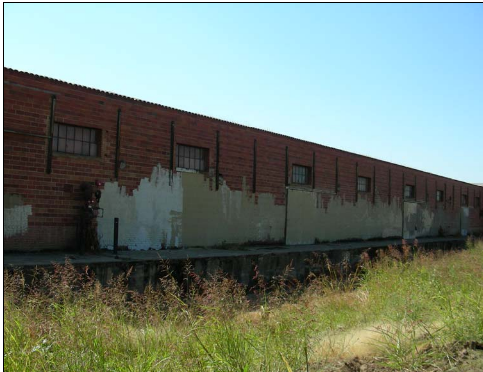
Photograph 23: Building 7, camera facing southeast, 08/29/2006.
