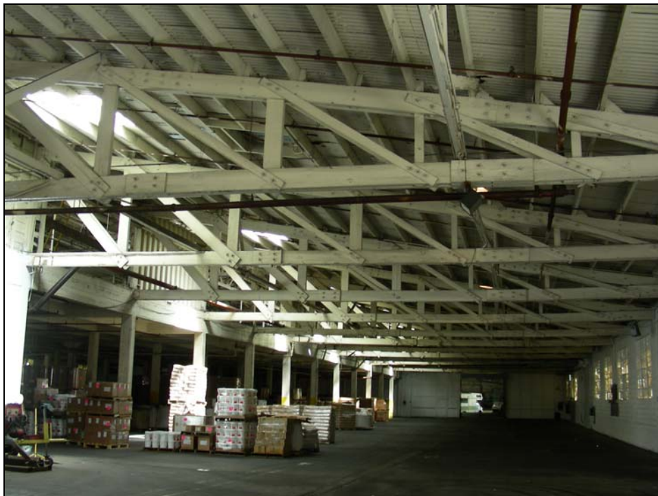
Photograph 15: Building 3, interior view of rafter construction and skylights, camera facing north, 08/29/2006.
