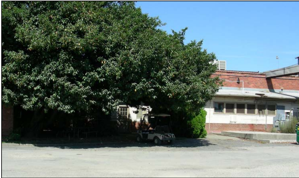
Photograph 32: Building 12, cafeteria, camera facing west, 08/29/2006.
