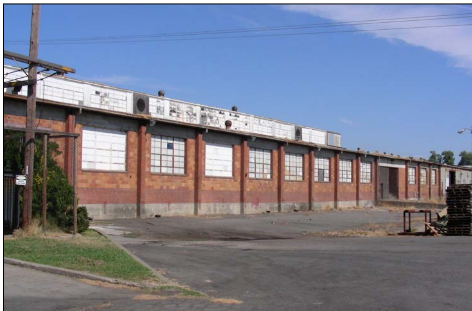
Photograph 12: Building 3, camera facing northwest, 08/29/2006.
