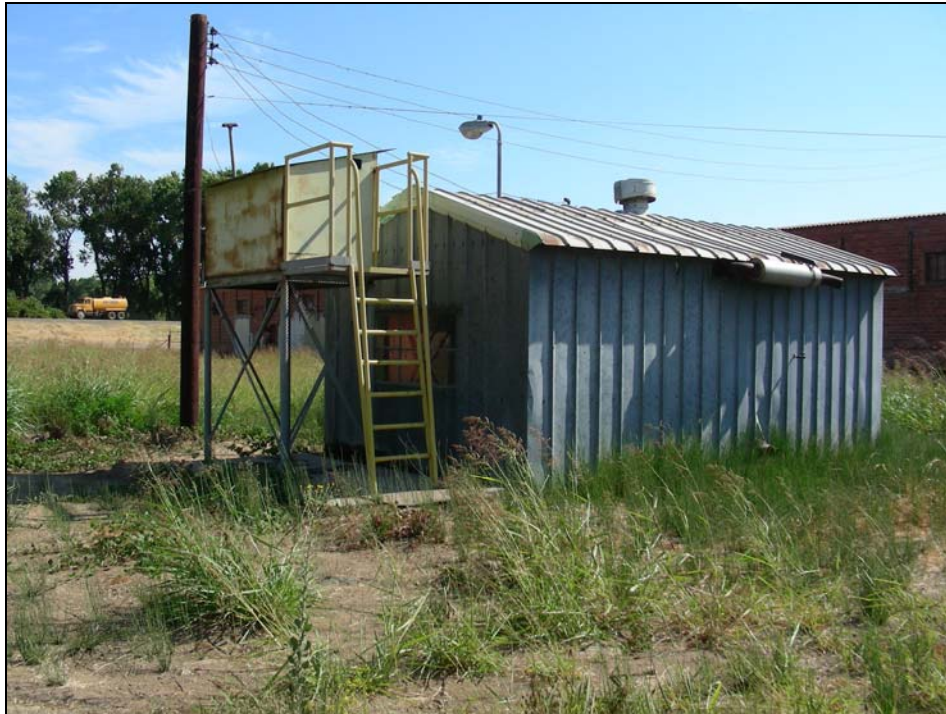
Photograph 36: Building 15, camera facing northeast, 08/29/2006.
