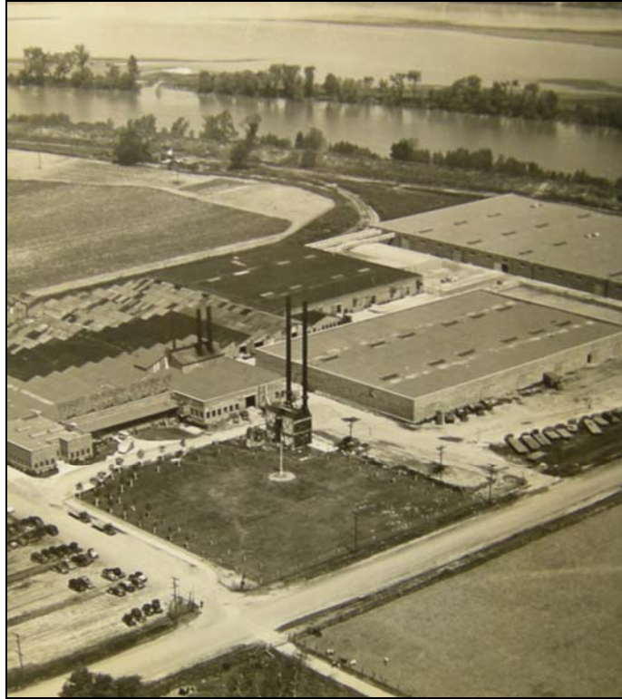
Photograph 1: Bercut-Richards Packing Company, ca. 1937. ( Sacramento Bee Photo Morgue, Available at SAMCC)
