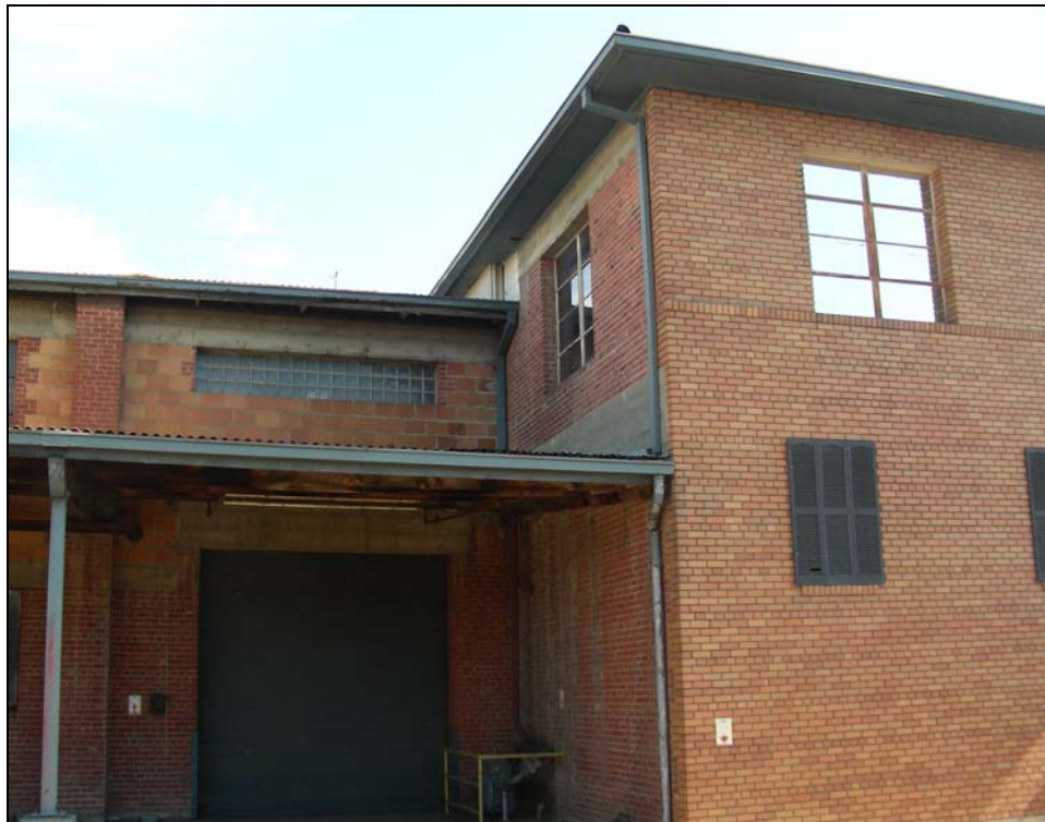
Photograph 9: Building 2 on left, Building 1 on right, camera facing north, 08/29/2006.
