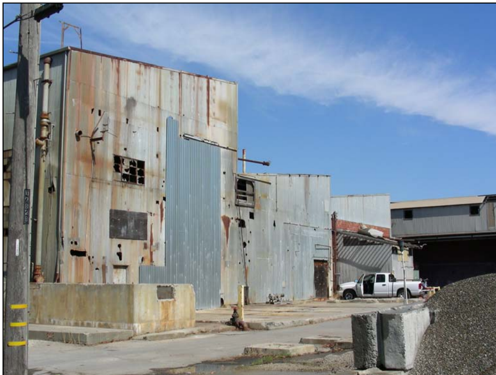
Photograph 19: Building 4, camera facing northwest, 08/29/2006.
