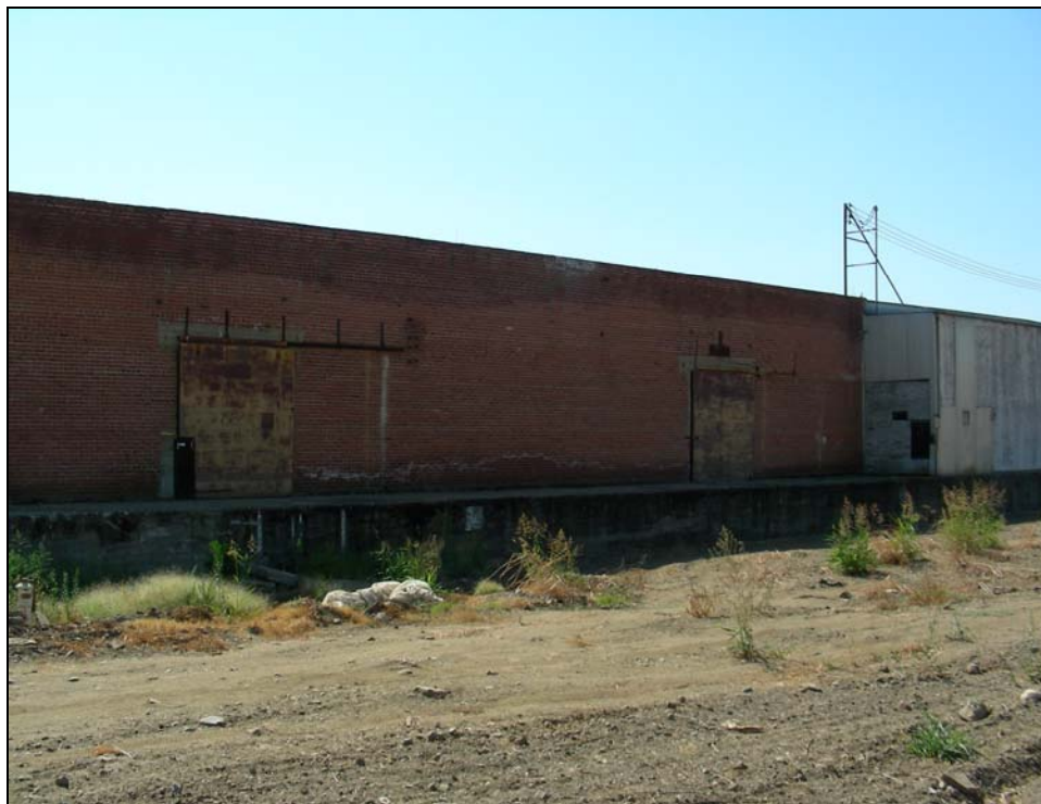
Photograph 21: Building 5, camera facing east, 08/29/2006.
