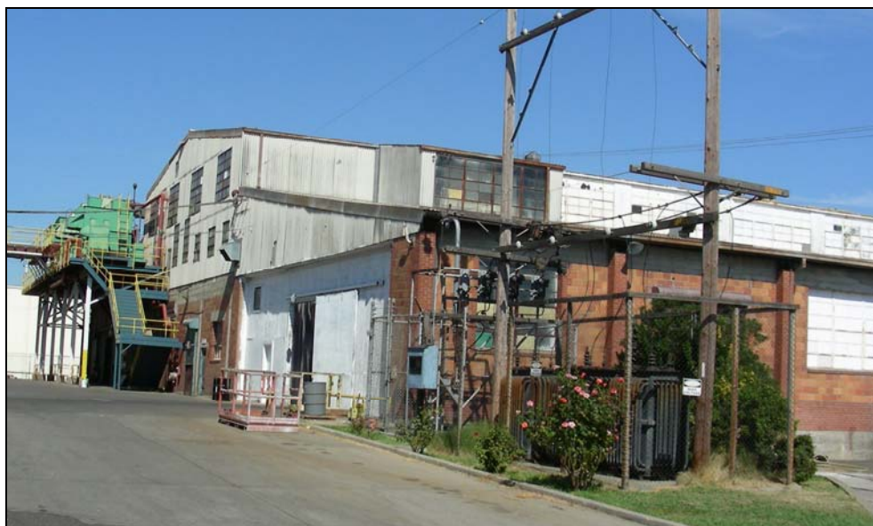
Photograph 13: Building 3, camera facing west, 08/29/2006.
