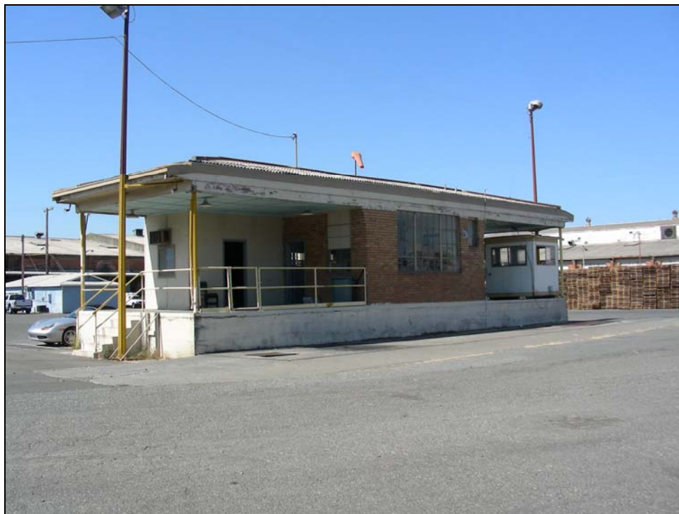
Photograph 30: Building 11, camera facing southwest, 08/29/2006.
