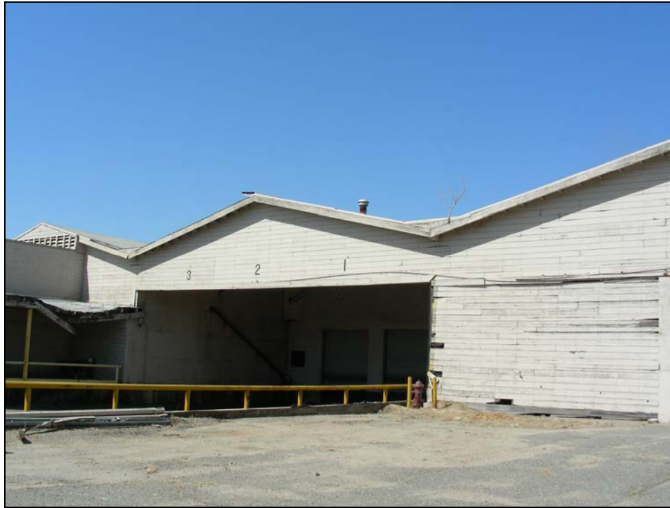
Photograph 22: Building 6, camera facing northwest, 08/29/2006.
