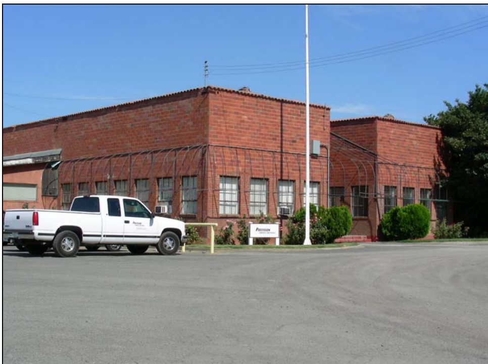
Photograph 31: Building 12, office building, camera facing northwest, 08/29/2006.
