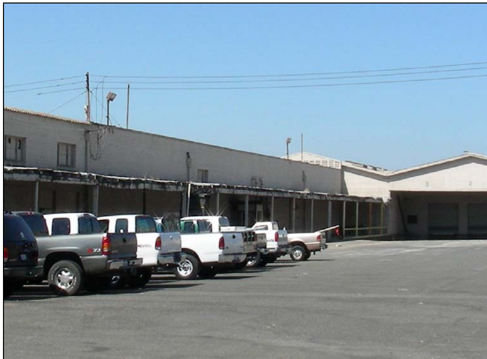
Photograph 27: Building 9, camera facing southwest, 08/29/2006.
