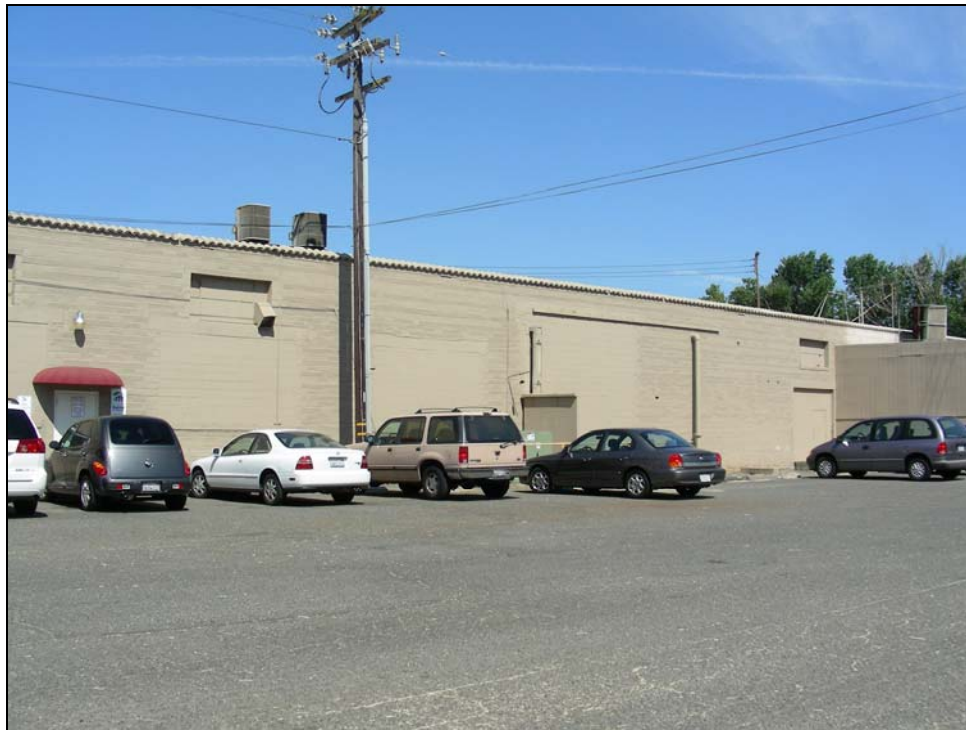
Photograph 26: Building 8, camera facing northwest, 08/29/2006.
