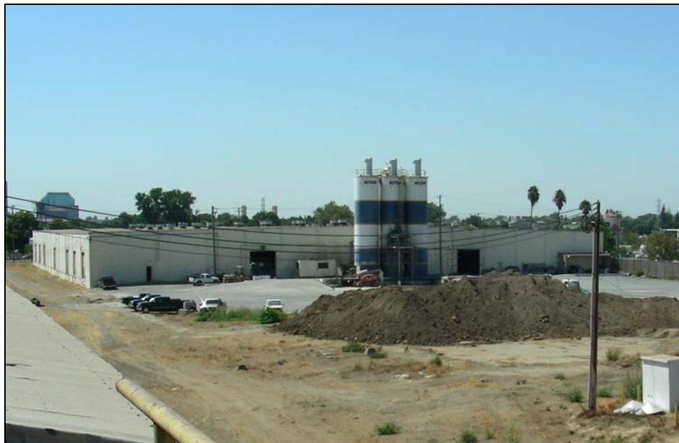
Photograph 35: Building 14, camera facing southwest, 08/29/2006.
