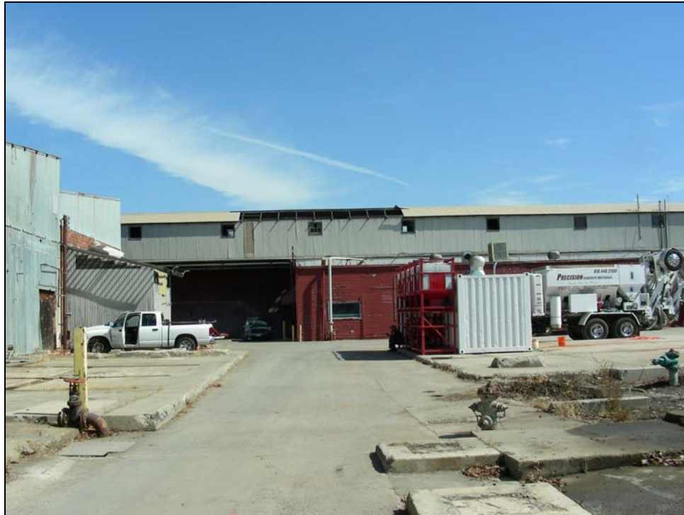
Photograph 28: Building 9, camera facing north, 08/29/2006.
