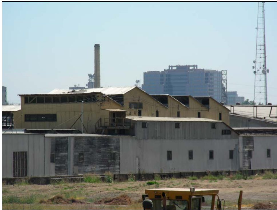
Photograph 16: Building 4, camera facing southeast, 08/29/2006.
