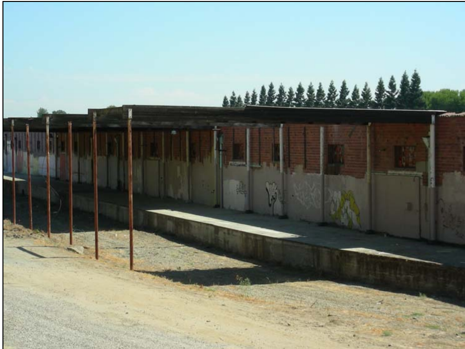
Photograph 24: Building 7, camera facing southeast, 08/29/2006.
