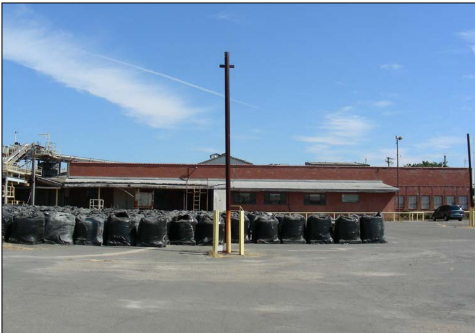
Photograph 33: Building 12, camera facing north, 08/29/2006.
