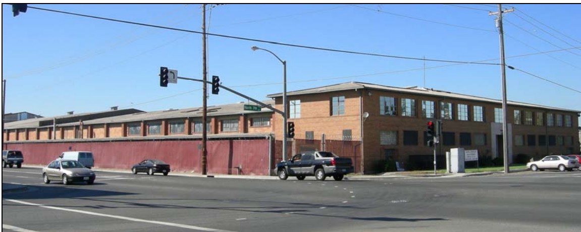
Photograph 4: Building 1 and 2, camera facing northwest, August 2006.
