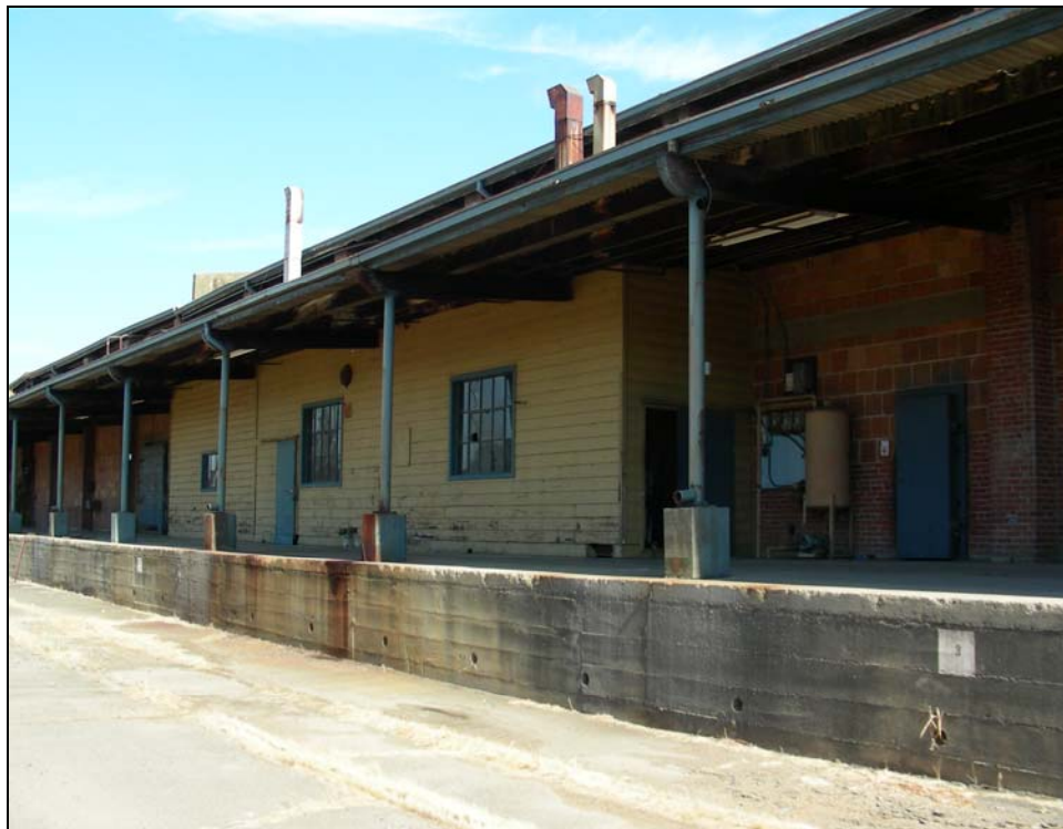
Photograph 11: Building 2, detail of loading dock on south side, camera facing northwest, 08/29/2006.
