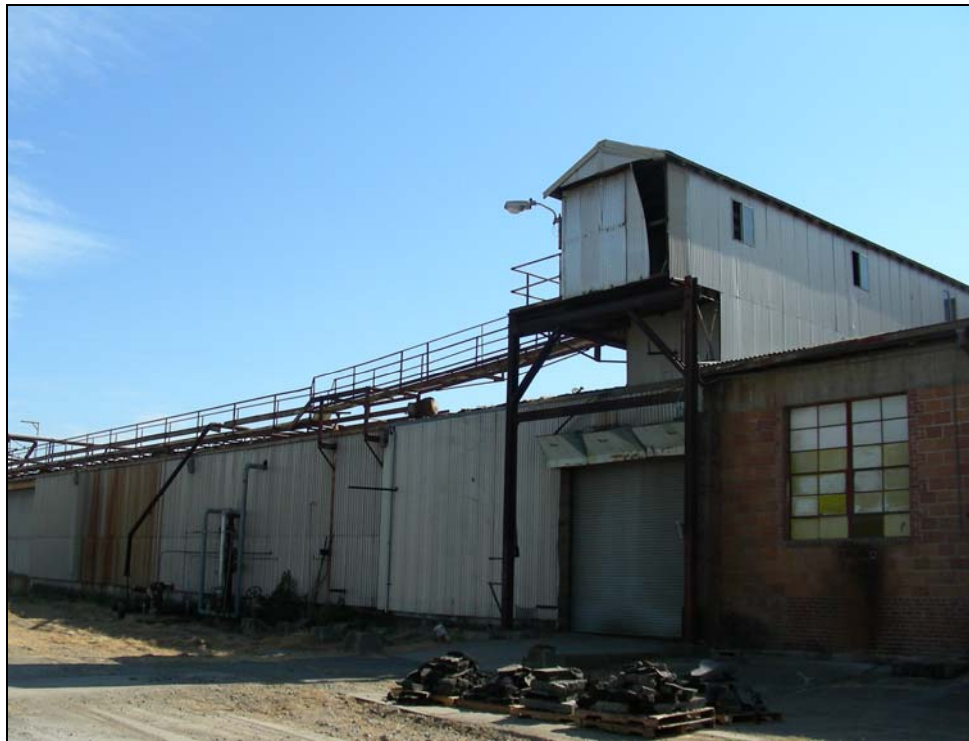
Photograph 20: Building 4, camera facing northeast, 08/29/2006.
