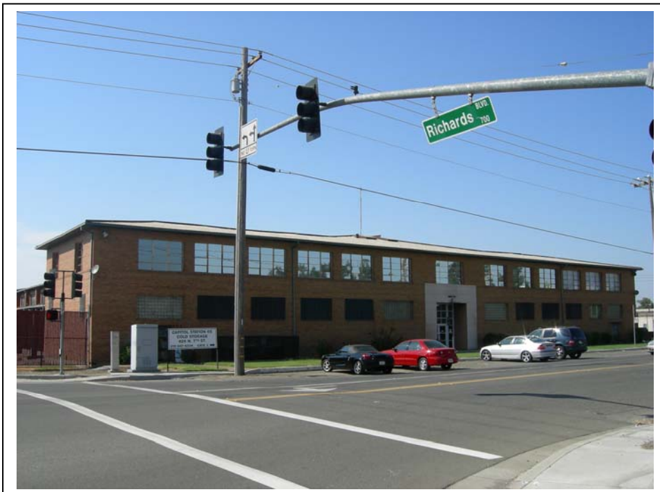
P5b. Description of Photo: (View, date, accession #) Photograph 1: Building 1, camera facing northwest, 1 September 2006.
