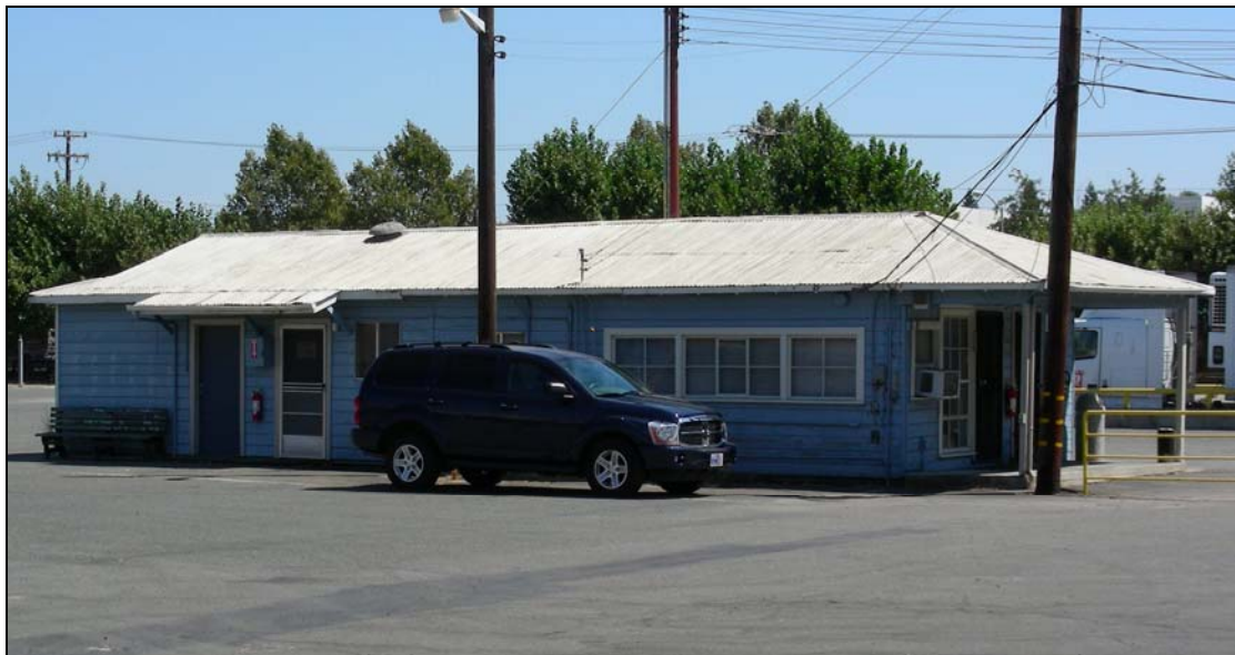
Photograph 37: Building 16, camera facing northeast, 08/29/2006.
