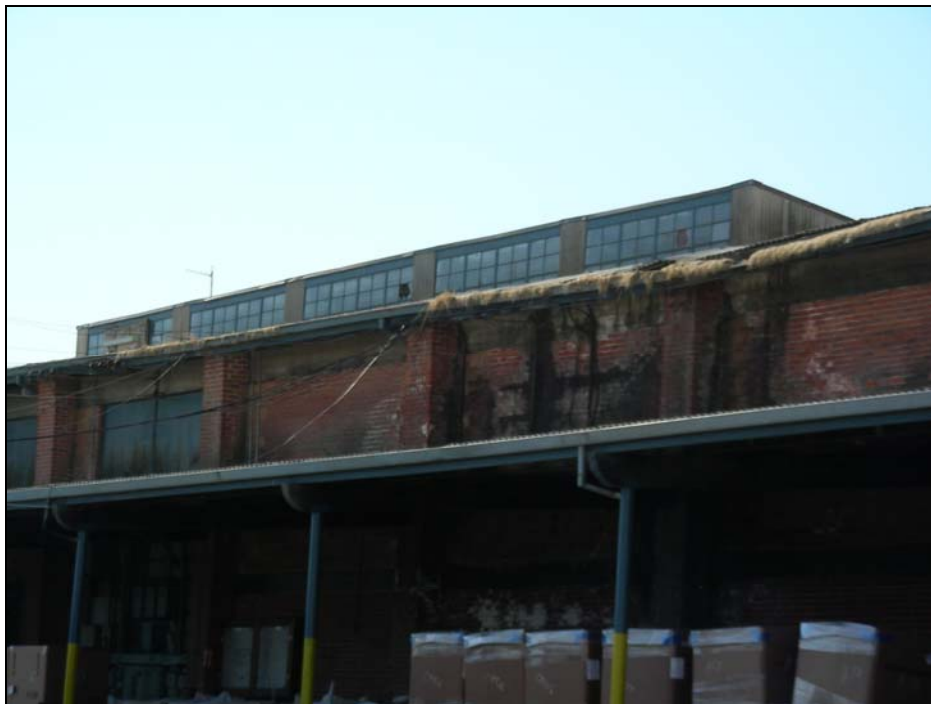
Photograph 7: Building 2, detail showing shed dormer, camera facing southeast, 08/29/2006.
