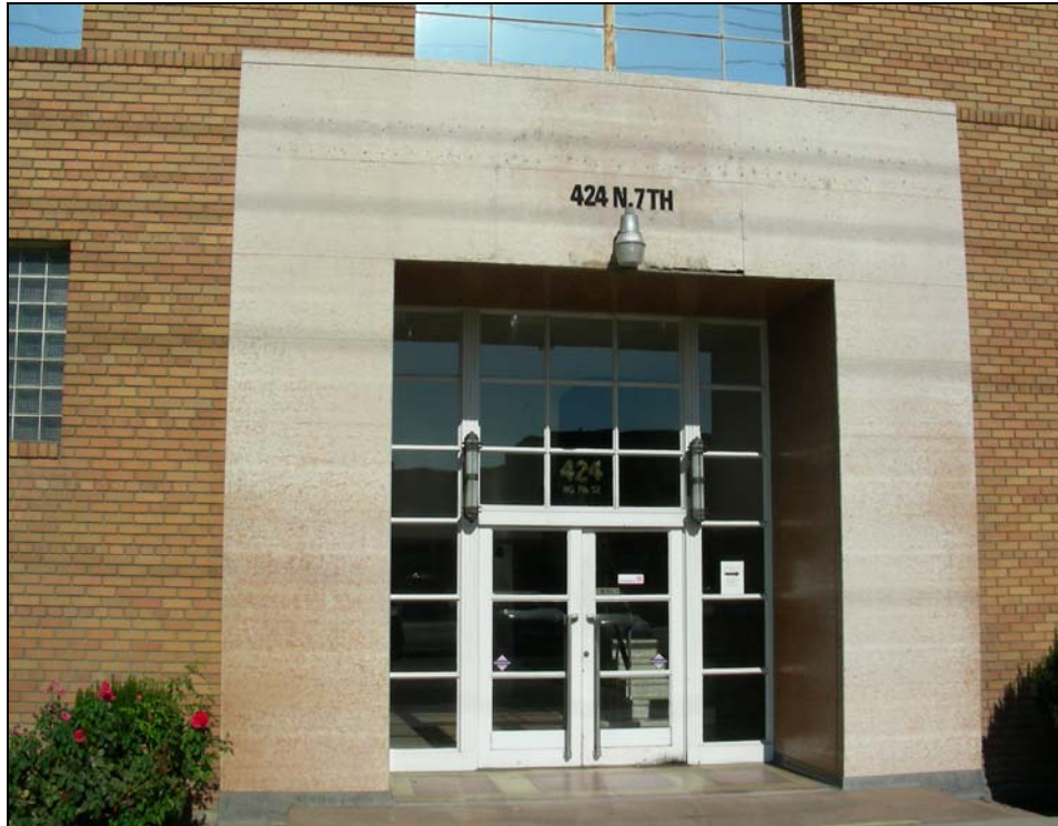
Photograph 2: 7 th Street Entrance to Building 1, camera facing west, 08/29/2006.
