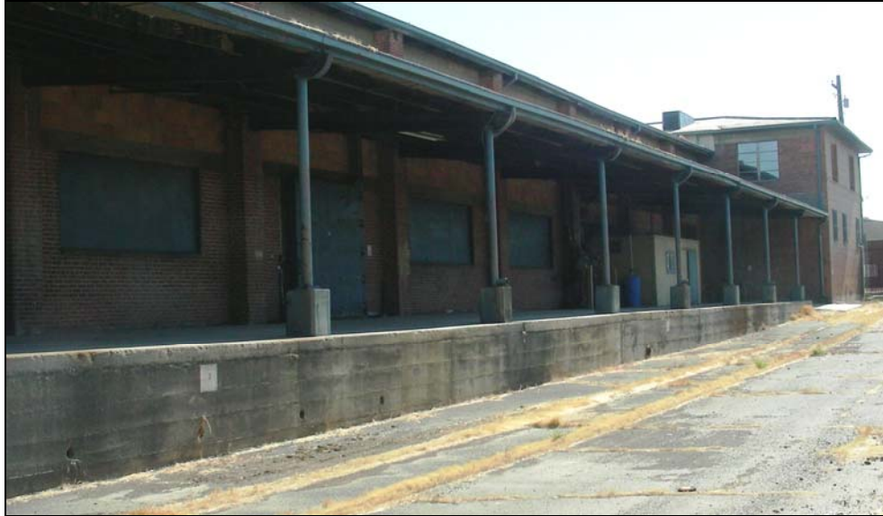
Photograph 10: Building 2, loading dock along south side, camera facing east, 08/29/2006.
