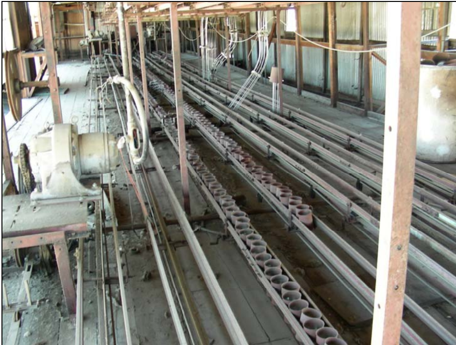
Photograph 18: Building 4, detail of can conveyor system, camera facing east, 08/29/2006.
