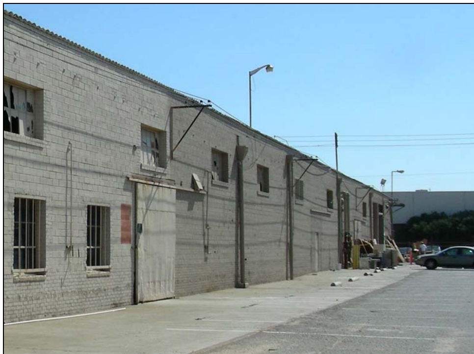
Photograph 25: Building 8, camera facing east, 08/29/2006.
