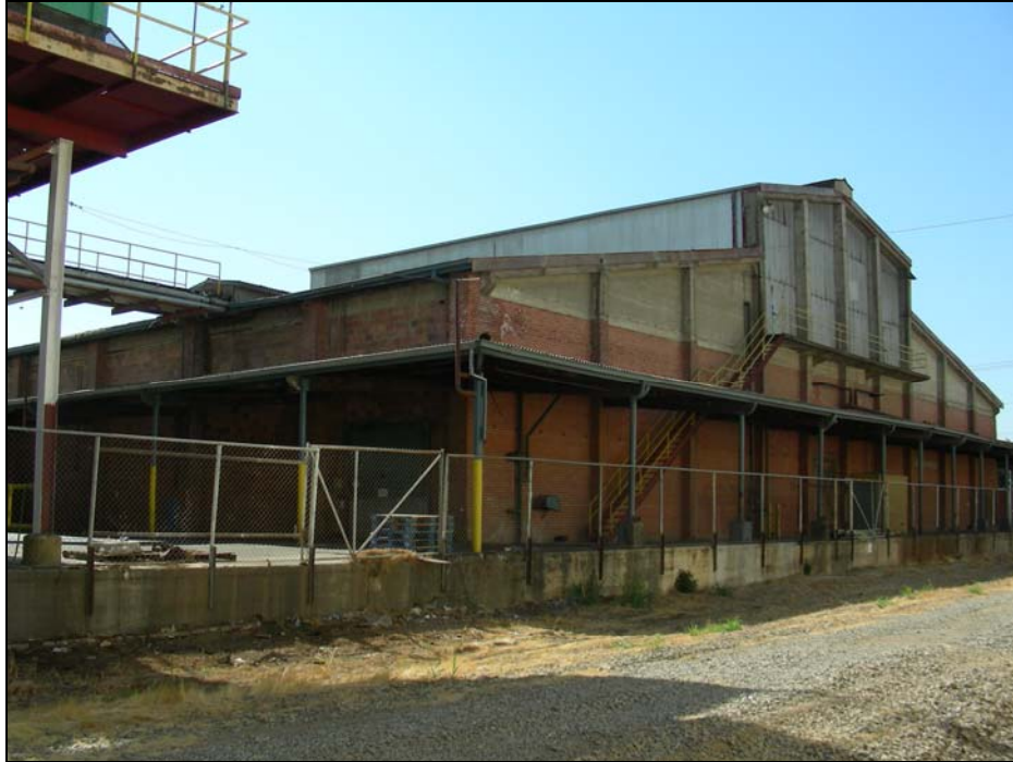
Photograph 8: Building 2, detail of monitor roof extension, camera facing southeast, 08/29/2006.
