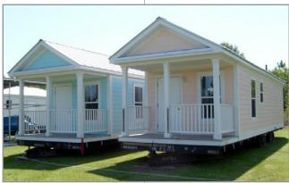
Manufactured Homes are required to have a wheeled chassis that is permanently attached
