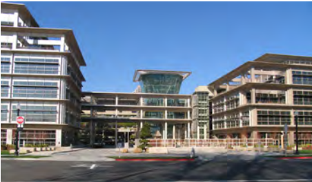
The CalPERS office building incorporates sustainable building practices.
