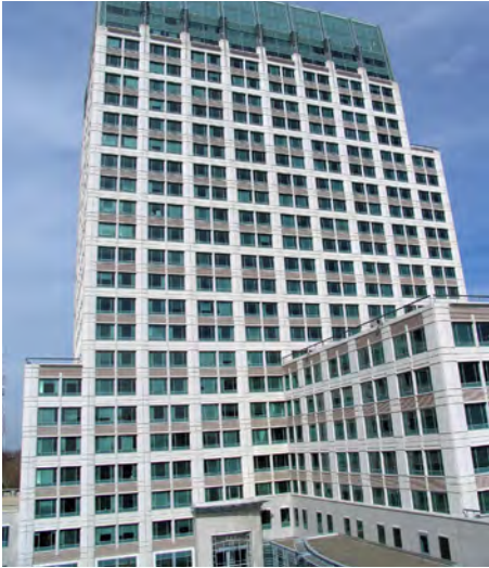
California Environmental Protection Agency Headquarters Building (Cal/ EPA) in downtown Sacramento became the first LEED for Existing Buildings Platinum certified building in 2004.
