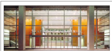
5 Building entrances that directly address the street and have a high degree of transparency
