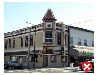
Figure 185. Many of the historic exterior features of this contributing building have been preserved and maintained; however, the windows and front facade have been partially covered by a ventilation duct.
