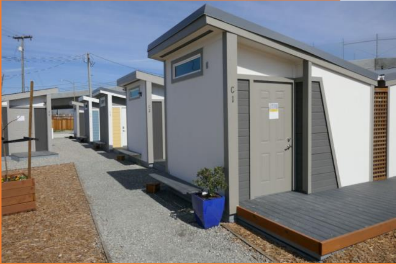
City of San Jose Housing Department
