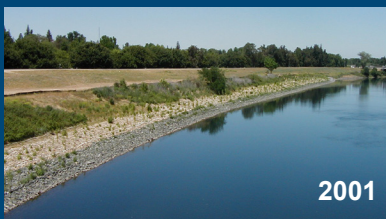
Erosion protection near CSUS with on-site mitigation completed in 2001
