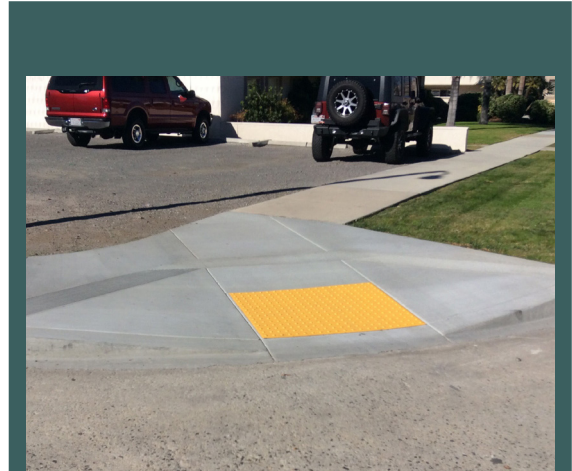
Compliant curb ramp
