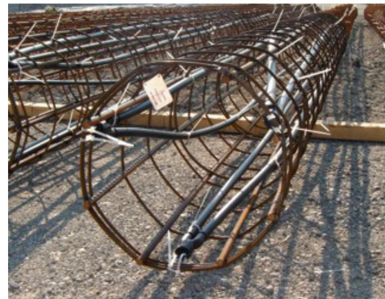
Figure 7.6 Ground Loop Tubing within Rebar Cages of Structural Piles
